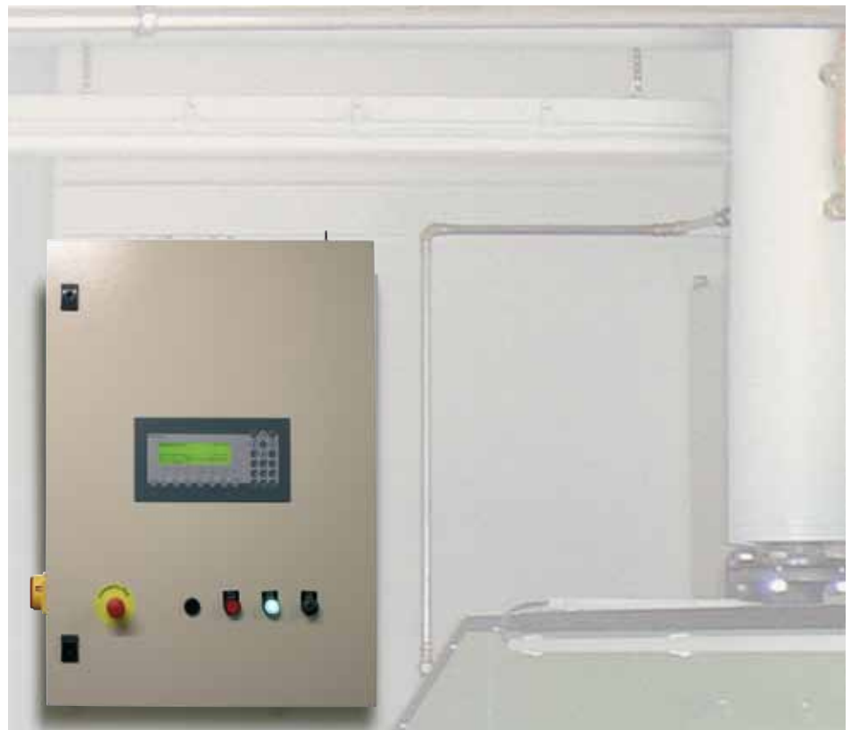
All components of the system are electronically controlled by a PLC controller inside the control cabinet. Current operating data from the combustion system is indicated on an illuminated display.
