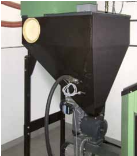
The intermediate container of the HDG pellet suction system can hold up to 100 kg of pellets.
